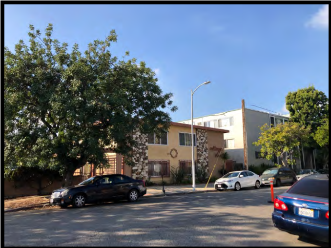
Photo #10: View of front of apartment to the northwest.
