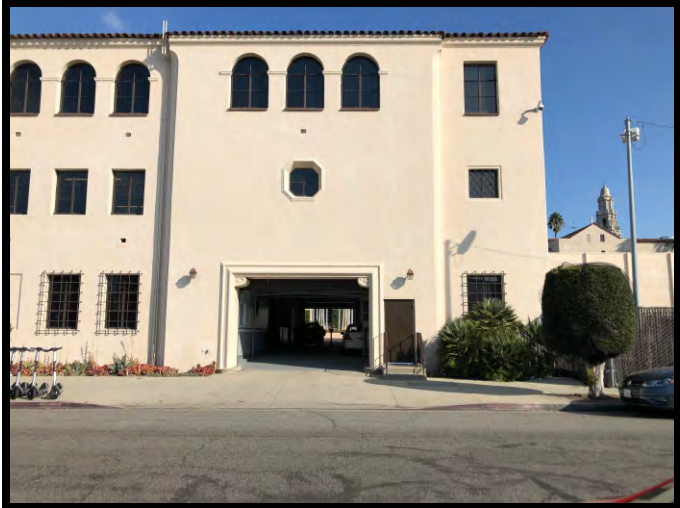
Photo #13: View of garage entrance on AAA property to northeast.
